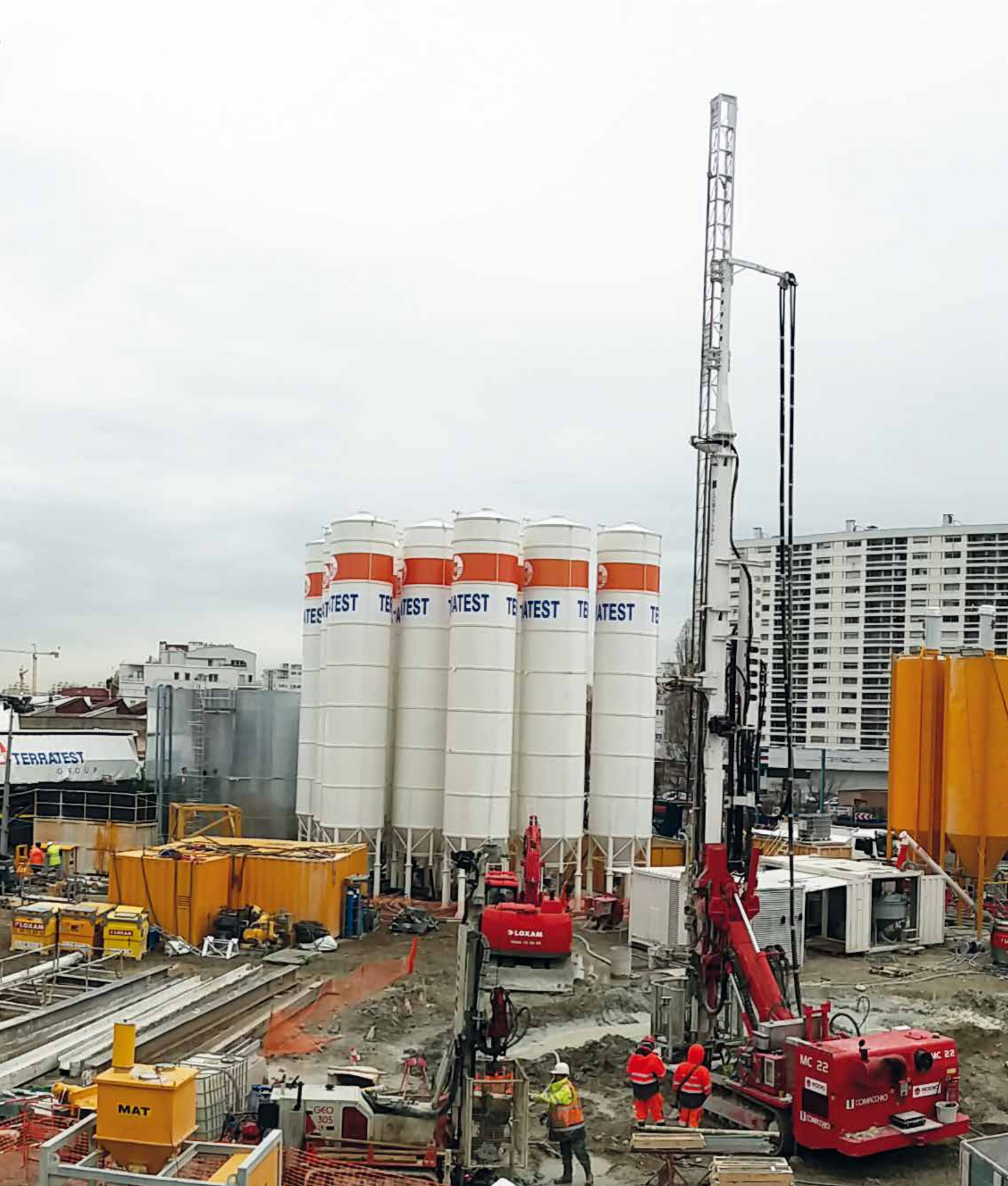
Grand Paris Express Line 16 (France) Diaphragm Walls, Grouting, Jet grouting and Bored Piles
