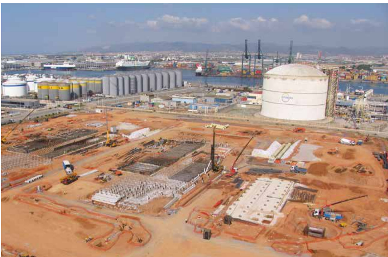
Gas Natural Combined Cycle Power Plant, Spain Precast Piles Corte Inglés Mall, Tarragona, Spain Diaphragm walls
