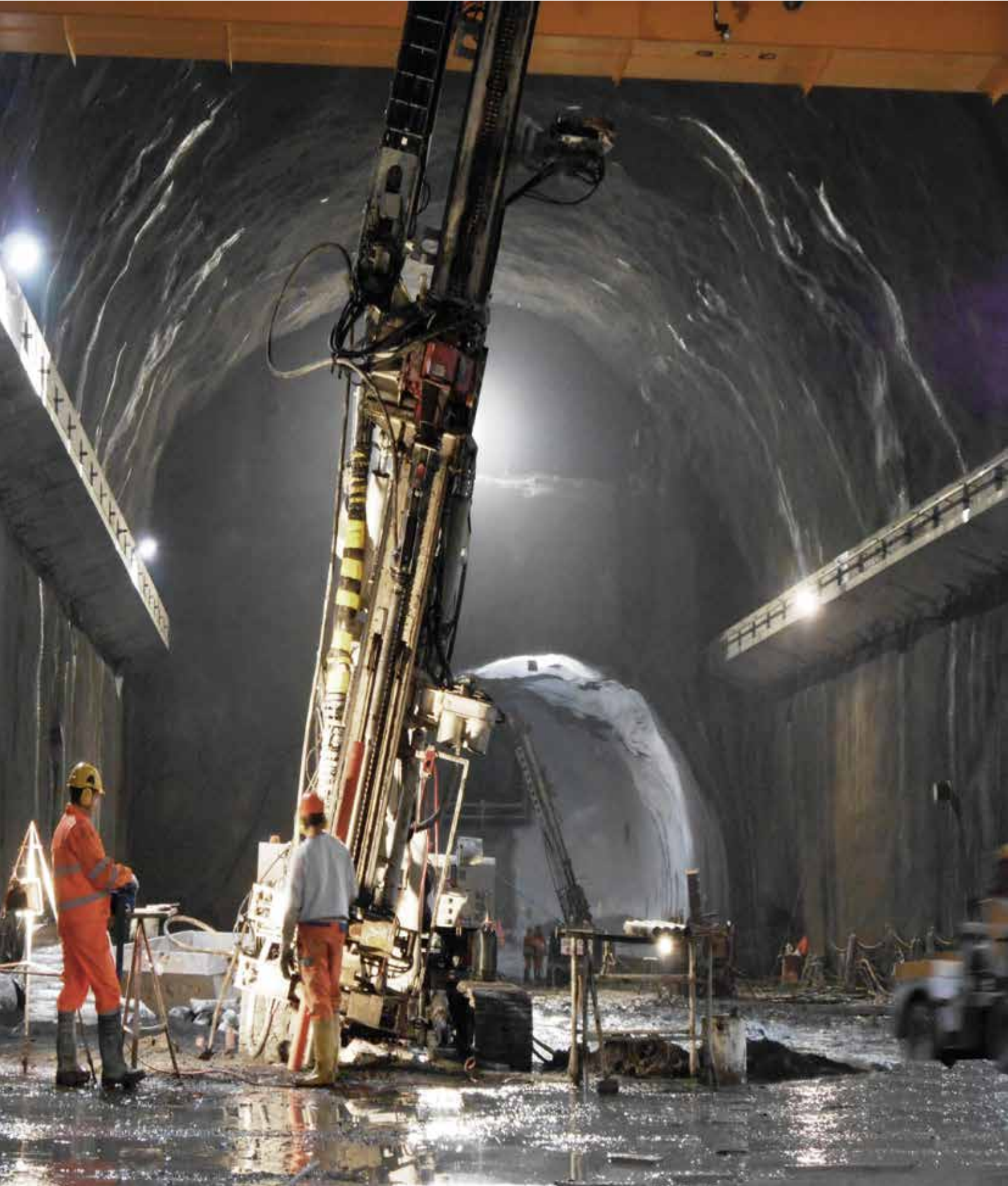
2ND Water Power Plant of Honggrin Léman Rock Grouting
