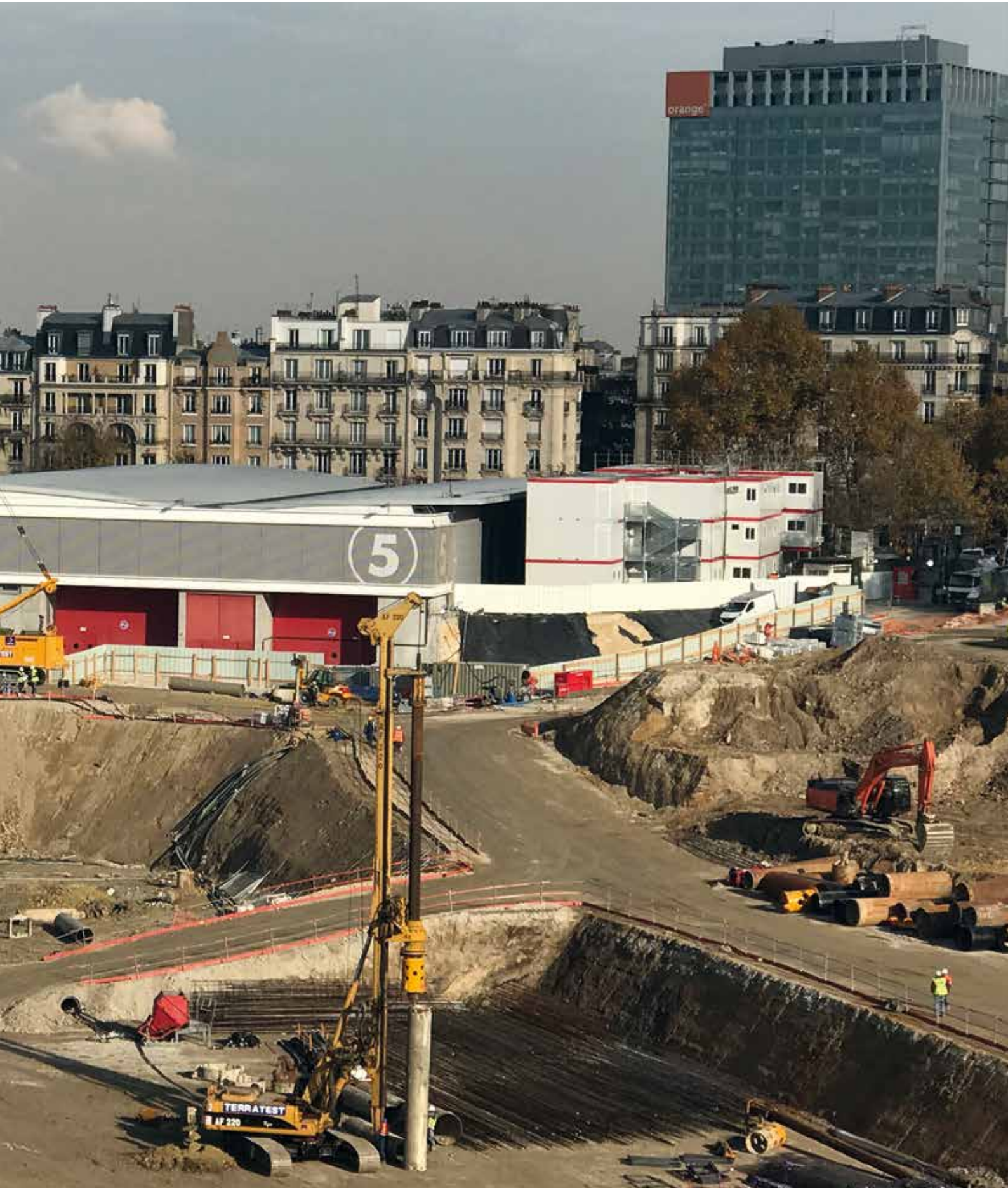
Paris Expo Porte de Versailles Convention Centre (France) Bored Piles
