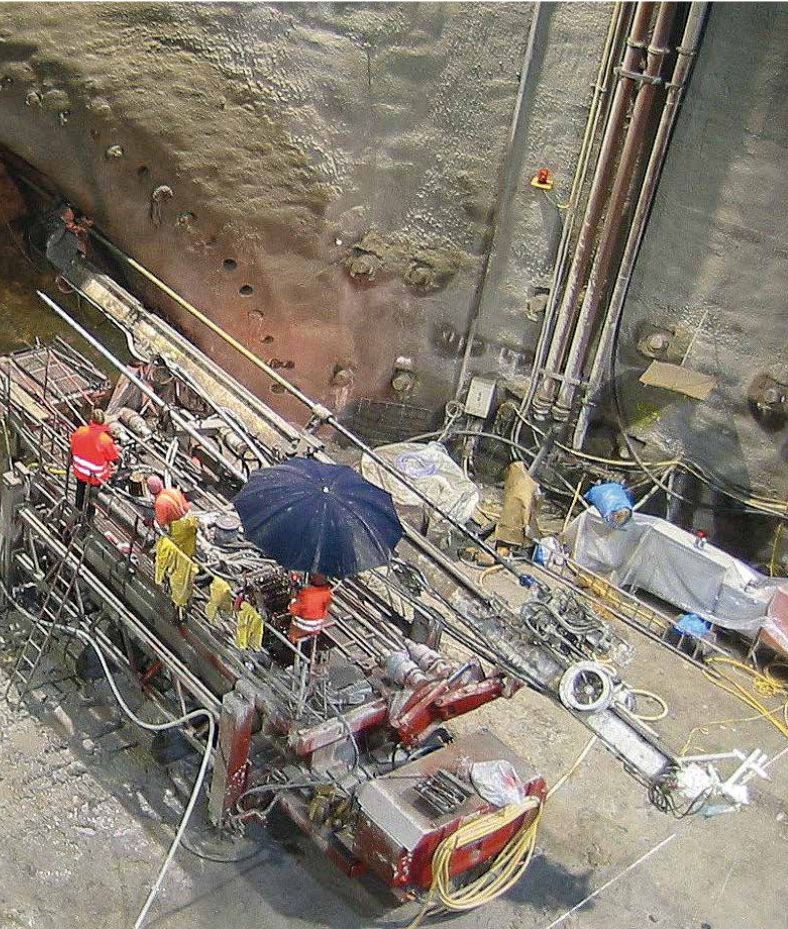
Tunnel U3 Olimpiapark Munich (Germany) Tunneling Works
