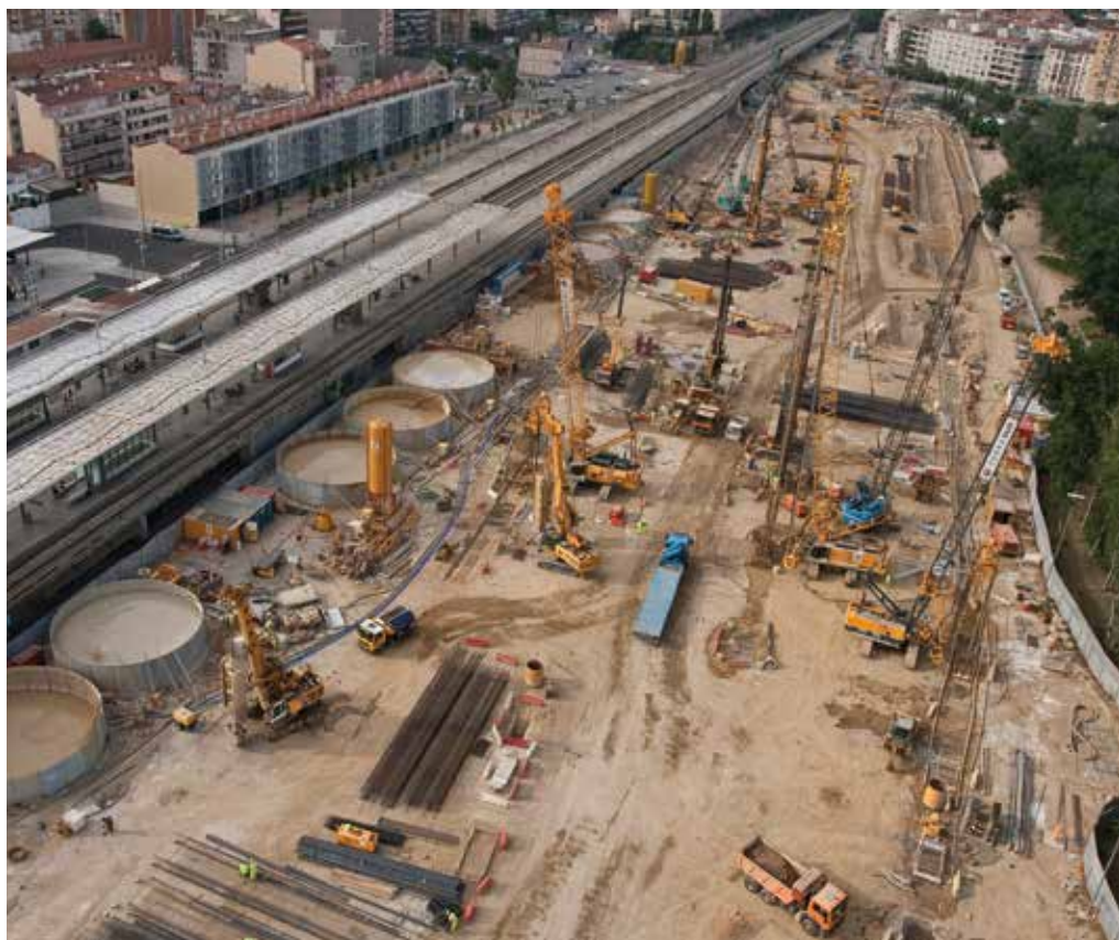
New High-speed railway station. Gerona, Spain Diaphragm walls, Bored Piles, Trench Cutter
