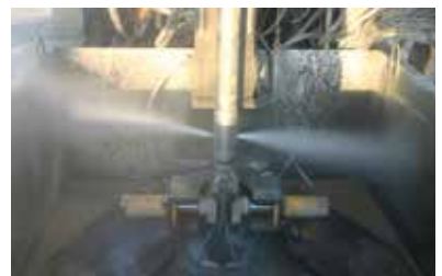
Compensation and Compaction Grouting
