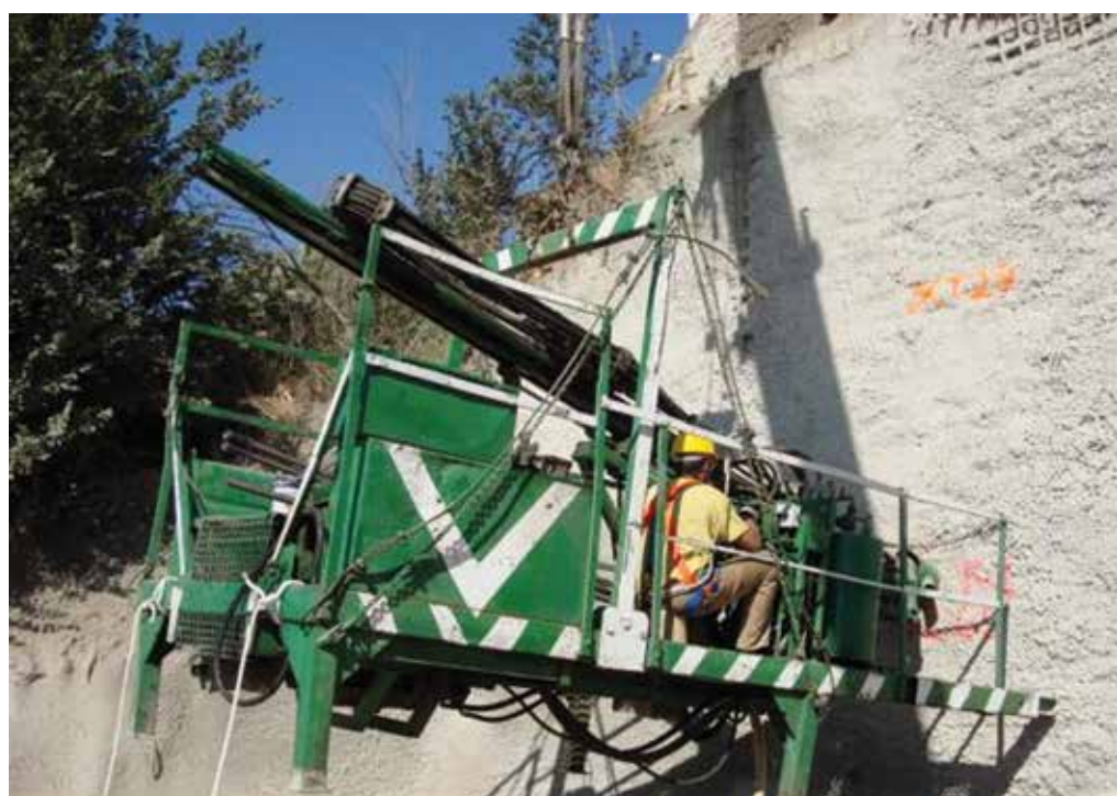
Landslide in Bonares. Huelva, Spain Soil Nailing
