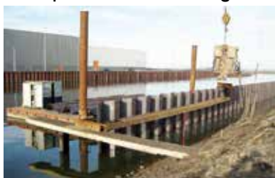
Sheetpiles / Metal Bracing
