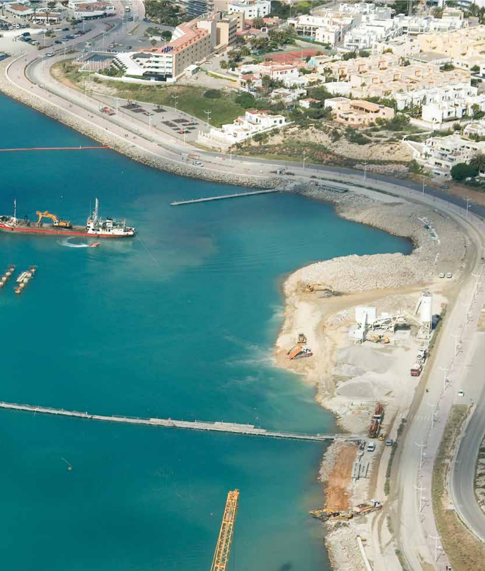
Botafoc Pier. Ibiza Port, Spain Bored Piles
