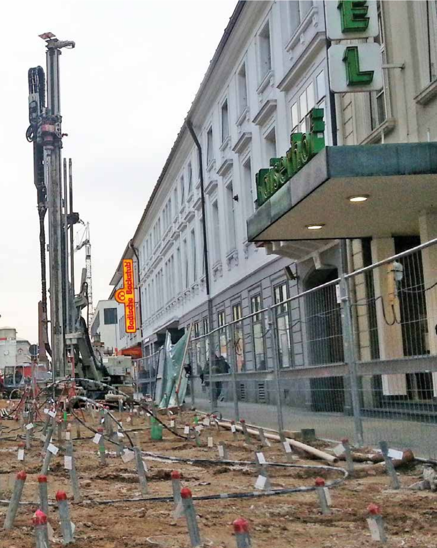
City Metro Tunnel Karlsruhe Manchette Pipe Grouting (Germany) Grouting
